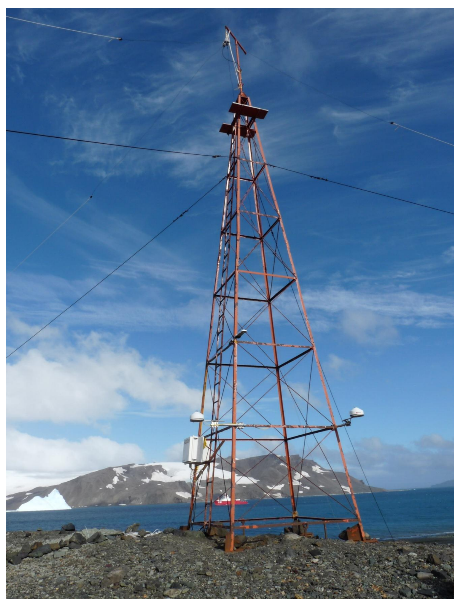
Fig. 5: Southeast view of the 12 meter South Tower instrumented with radiation sensors.
